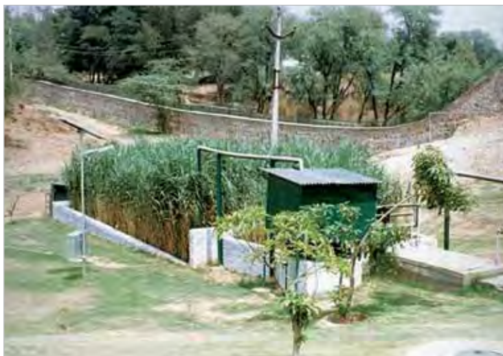
Figure 7 Root zone system for waste water treatment
