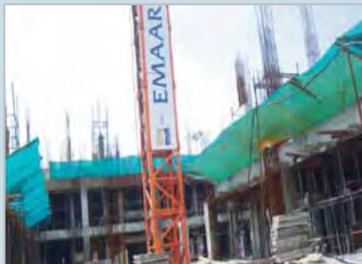
Figure 4 Safety nets at construction site
